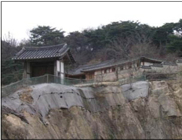
Figure 11. Damaged the original form to Seokpajeong Garden in 2006[23]
