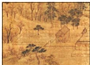
Figure 5. Byeoldang Villa and pond
