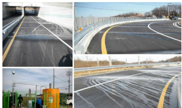
Fig. 2 Roadside Spray Type and Median Spray Type
