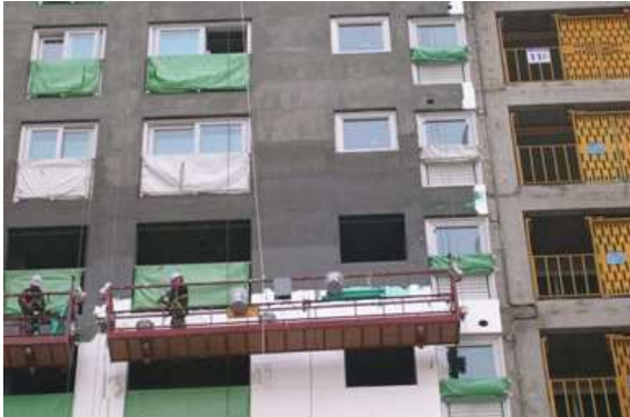
Figure 2. EIFS work using gondola
