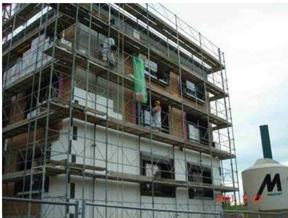
Figure 3. EIFS work using scaffold
