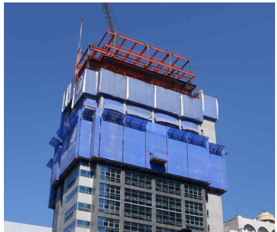
Figure 4. EIFS work using auto climbing platform
