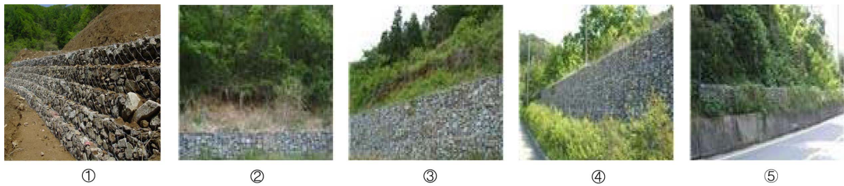
Figure 1. Photographs provided to scenic preference analysis of gabion; ① Scenic view following gabion works in cutting slope of roads, ② Scenic view following seed spray sowing between gabion works, ③ Scenic view following herbaceous vegetation sowing under gabion, ④ Scenic view following 50% screening by shrub planting under gabion, ⑤ Scenic view following screening by runner plants on gabion.
