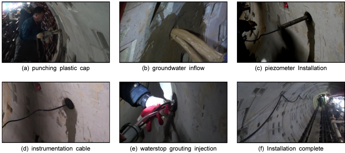
Fig. 12. Installation process of piezometer
