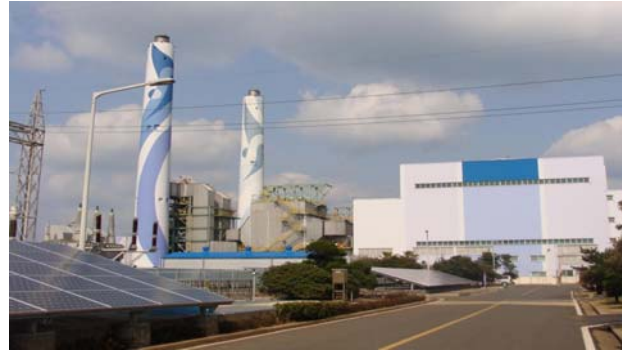
Figure 1: Thermal power plant
