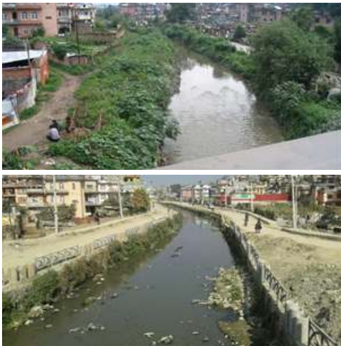
Fig. 7 River section before and after the river management at Kalopul (2005 and 2014)
