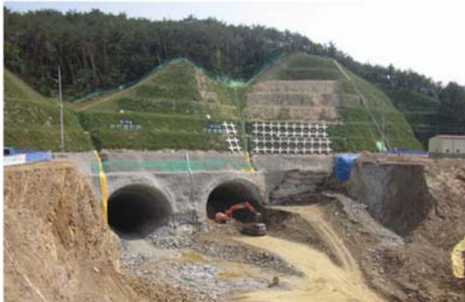
Fig. 23. Site landscape after ultimate remediation using grid anchor-blocks and tunnel grouting.
