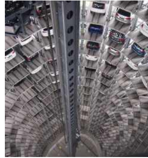
(Figure 7) AUTOSTADT Car Tower
