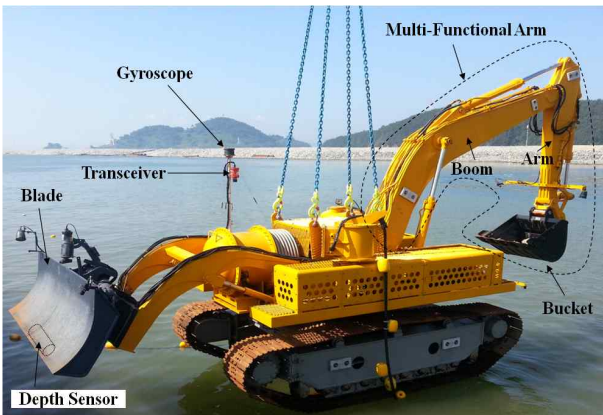
Fig. 1 Underwater construction robot for rubble leveling
