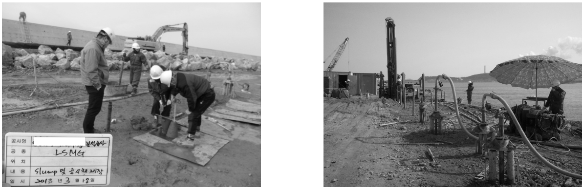
Fig. 8. Slump test (left) and LSMG execution (right)
