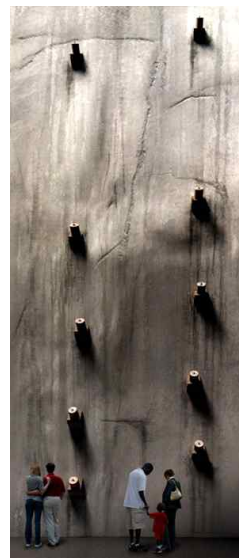
fig 8 WTC slurry wall © Studio Libeskind
