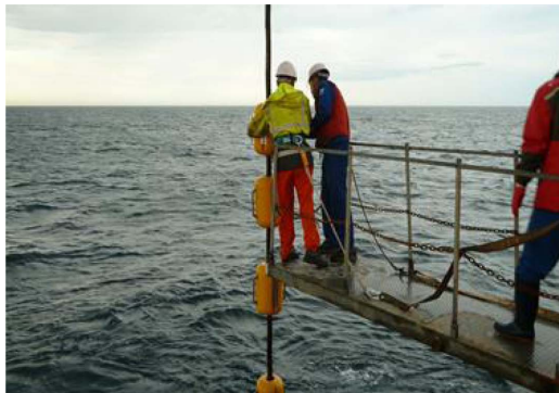
Fig. 2. Installation experiment of buoyancy module in real sea
