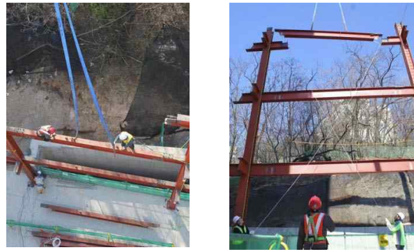
1. (a) conventional method 2. (b) DFA technology Figure 2. Comparison of fabrication method [12]
