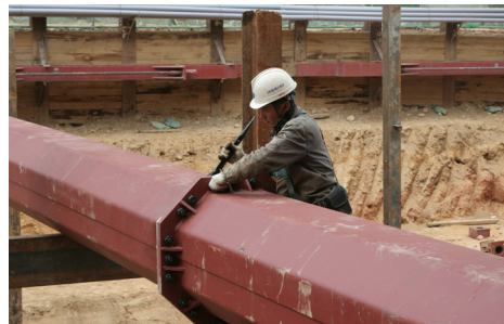
Fig. 2. Splice of OHS at mid point
