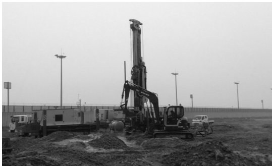
(a) Drilling of borehole
