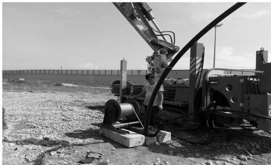
(c) Installation of GHE pipe and grouting (geohil)
