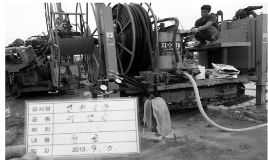
(b) Installation of GHE pipe and grouting (vertical closed loop)
