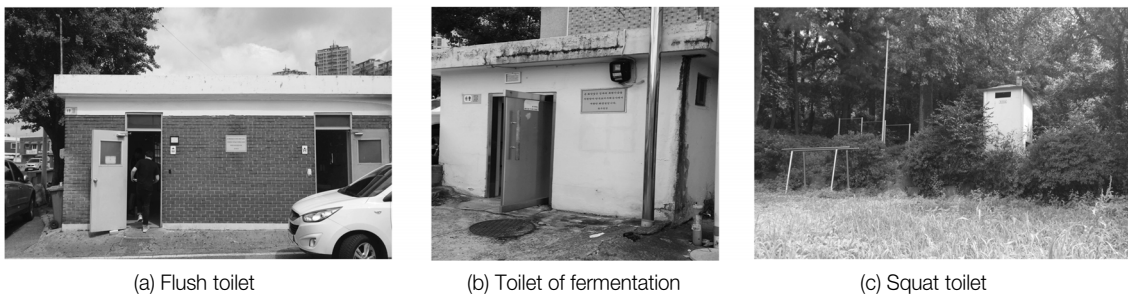
Fig. 1. Photos of public toilets by the way of handling.
