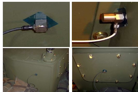
Fig. 9 Acceleration sensor at turret structure
