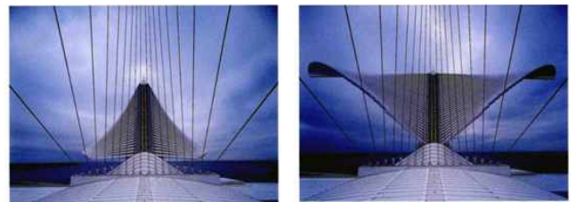
Fig. 15. Pictures of the Brise Soleil
