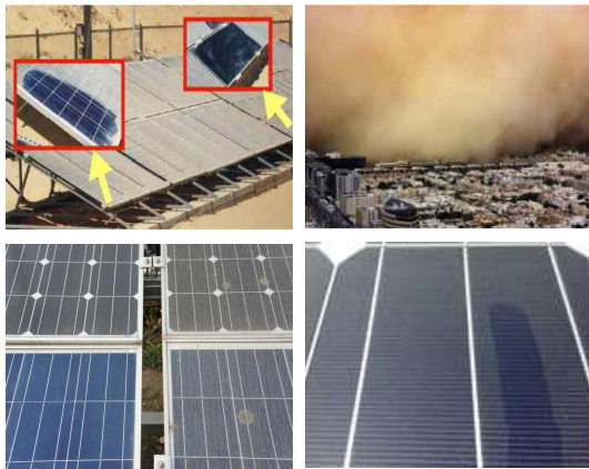
Fig. 1. Dust layer accumulation on PV modules in desert (top left) 5) , sand storm (top right) 6) , comparison with cleaning and non-cleaning modules in Bangladesh (bottom left), and yellow dust in Korea (bottom right)
