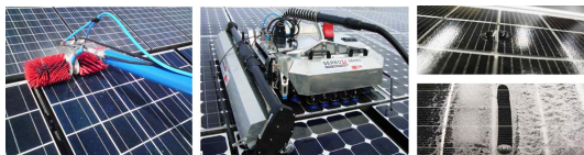
Fig. 12. Cleaning methods: water spray (left), self-cleaning robot (middle), hydrophobic coating (right) 5)
