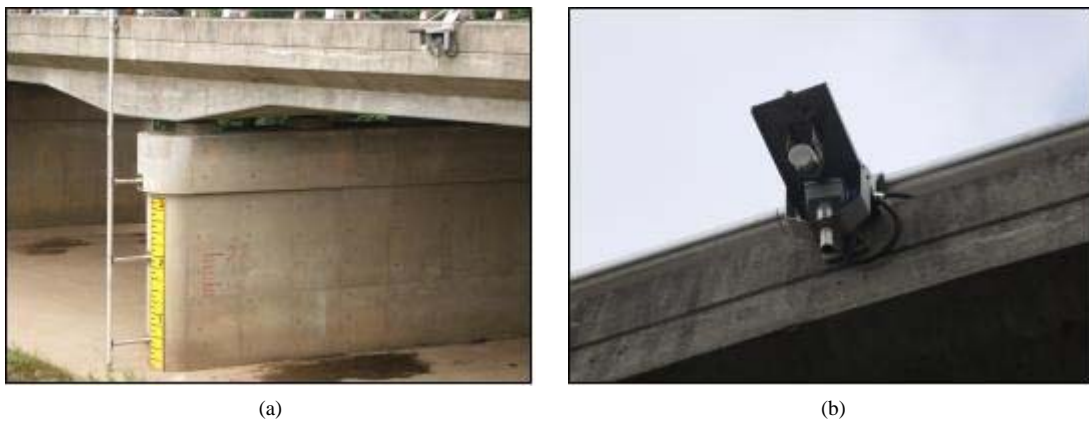
Fig. 7. Kalesto installed at Seong-eup bridge.
