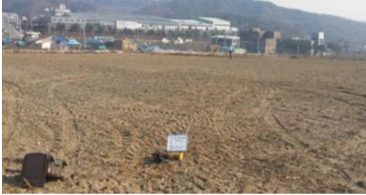
Fig. 6. Measurement of Ground resistance in Construction site
