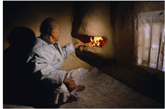
Figure 5. Kokeul Is an Interior Feature Which Functions Both as Heating and Lighting Device.
