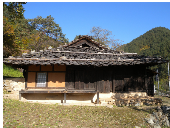
Figure 3. Neowa Houses with Full-Length Wooden Wall on the Right Side of the Facade. Source. Author
