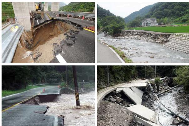
Fig. 3 Damage of Road and Embankment due to Heavy Rain and Typhoon
