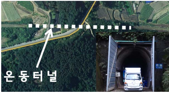
Fig. 1 Location and portal of test tunnel
