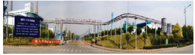
Fig. 2. 360m/10kA high-temperature superconducting DC cable [2].
