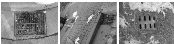
Fig. 6. Types of Rainwater Drainage
