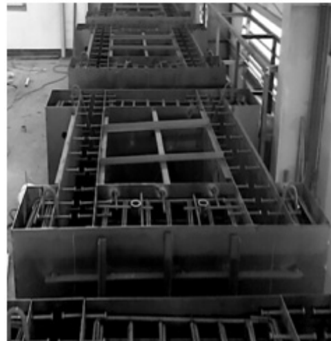
Fig. 3. Steel Plate Form Work
