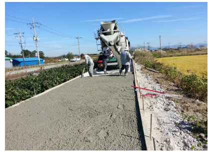
(c) Cast-in-place concrete
