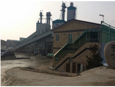
(a) Views of ready-mixed concrete plant
