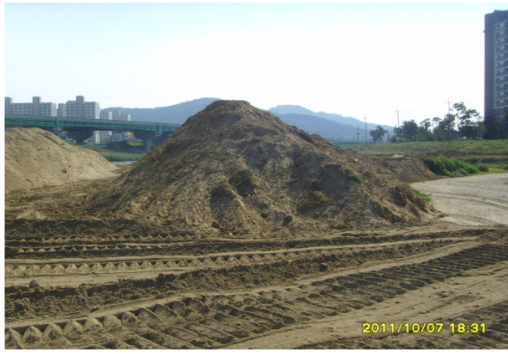
(a) Stockpiling topsoil
