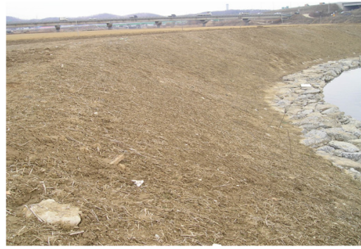
(b) Spreading topsoil
