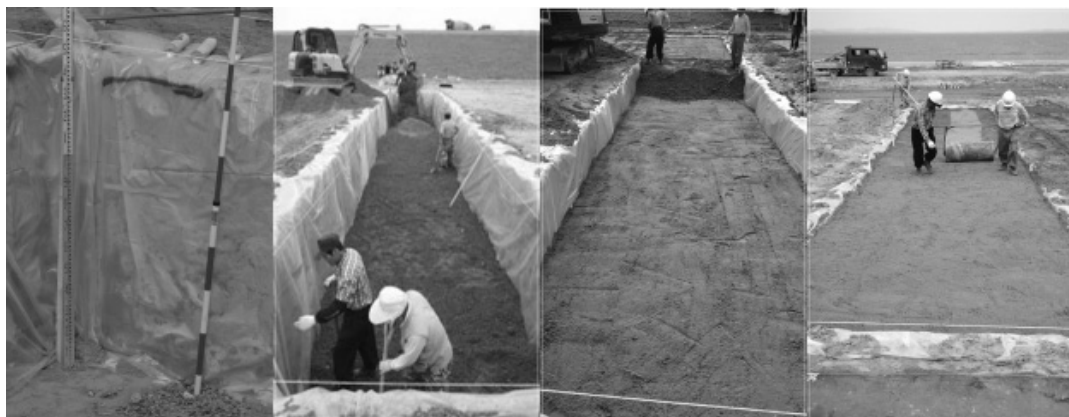
Figure 2. Construction processing of drainage layer for study plots.
