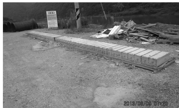
Fig. 2. Form work of test pieces.
