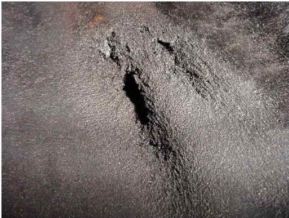
Fig. 2. Damaged surface by LDIE.
