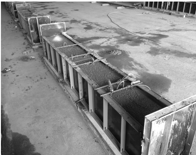
Fig. 7 Match casting
