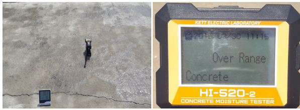
(a) Humid surface treatment (b) Concrete moisture testing
