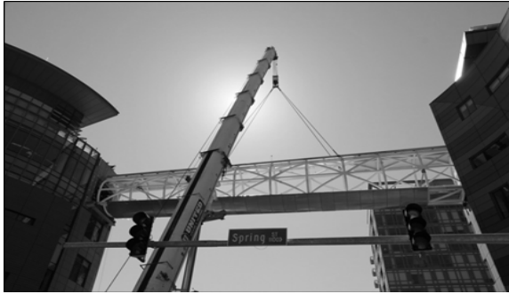
Figure 4 The connector bridge was installed on March, 11, 2012
