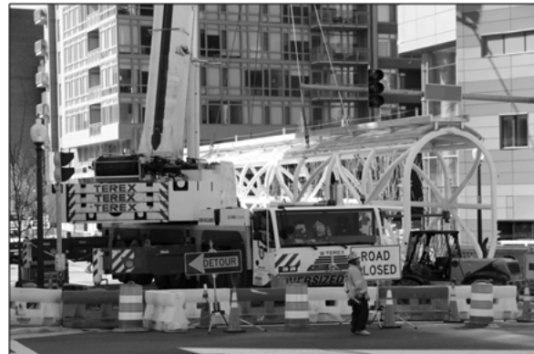
Figure 14 Actual site logistics after following the site logistics plan developed using BIM
