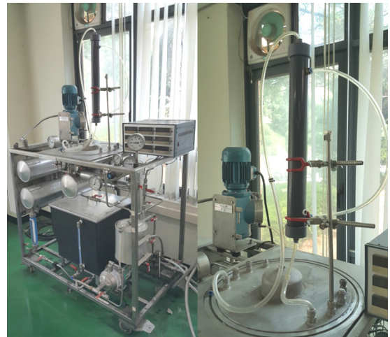
(A) Pilot test equipment (B) Membrane
