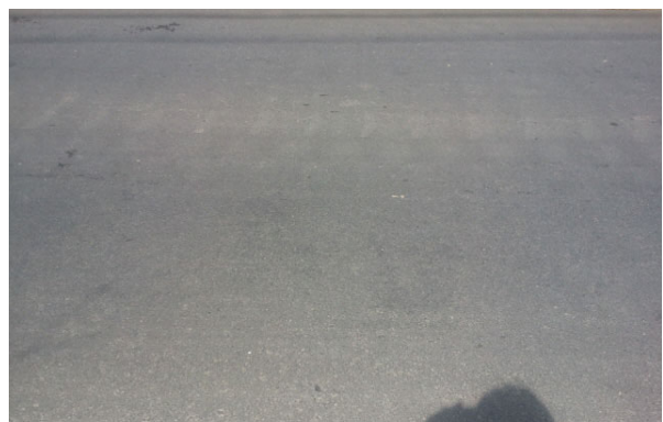
Fig. 8 Surface Condition using Micro-Surfacing in NH30
