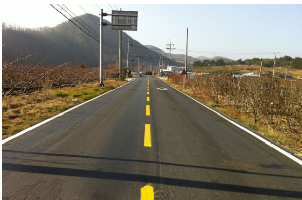
Fig. 11 Surface Condition using Polymer Slurry Seal in NH34
