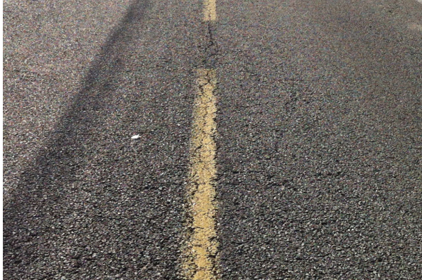
Fig. 9 Surface Condition of Existing Asphalt Concrete Pavement in NH34
