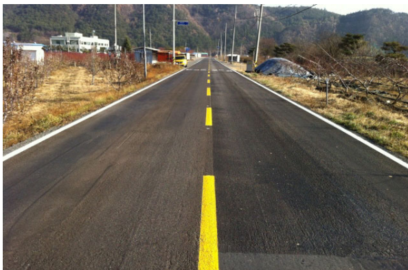
Fig. 10 Surface Condition using Micro-surfacing in NH34
