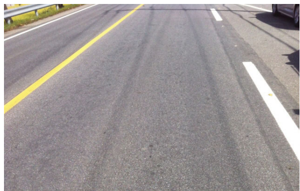
Fig. 7 Surface Condition using Polymer Slurry Seal Method in NH30
