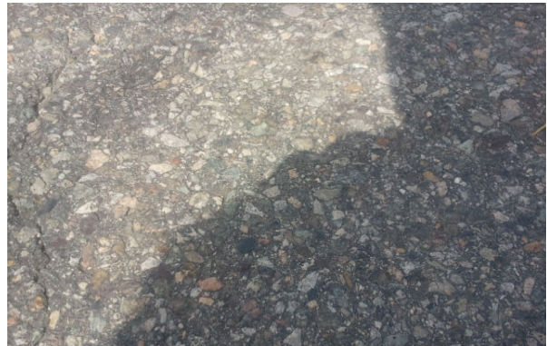
Fig. 6 Surface Condition of Existing Asphalt Concrete Pavement in NH30
