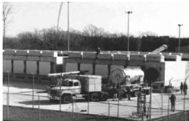
Fig. 4. Horizontal concrete module storage facility in Calvert Cliffs site [17].
