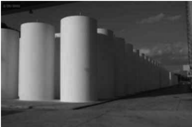
Fig. 5. Vertical concrete silo in Wolsong power plant site.
