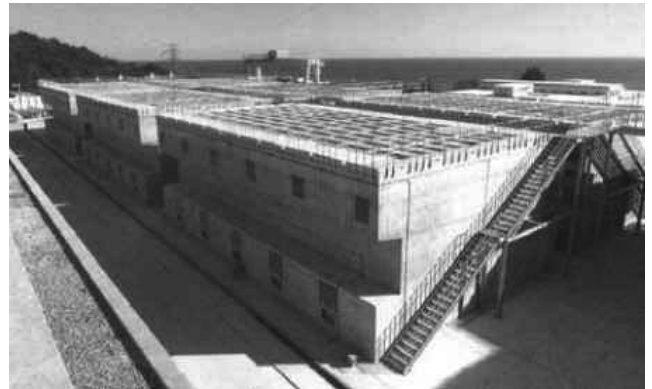
Fig. 6. MACSTOR-400 vertical concrete module in Wolsong power plant site [1].
