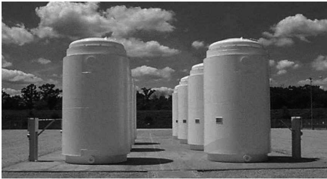
Fig. 8. Metal cask storage facility for spent fuel [20].
