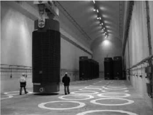
Fig. 10. Exterior and inside of the rock cavern storage facility in Neckarwestheim nuclear plant site [24].
