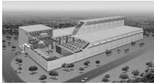
Fig. 9. Mutsu centralized spent fuel storage facility under construction [22].
