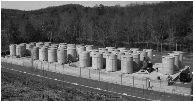
Fig. 7. Concrete cask storage facility in Connecticut Yankee power plant site [19].
