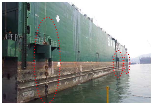
Fig. 10 Connections between floating dock and mooring chains (upper: starboard, lower: port)
