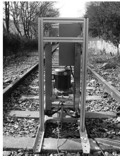
(b) Installation of penetrator
