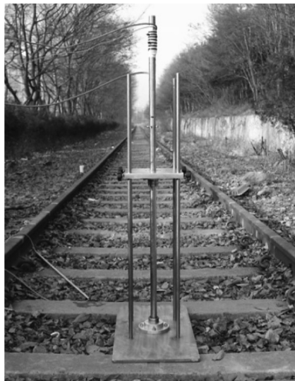
(a) Installation of guide
