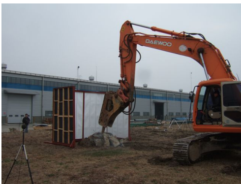
(b) After installation
