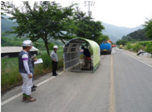
(b) After installation
