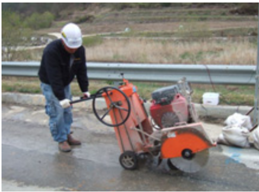
(a) Before installation
