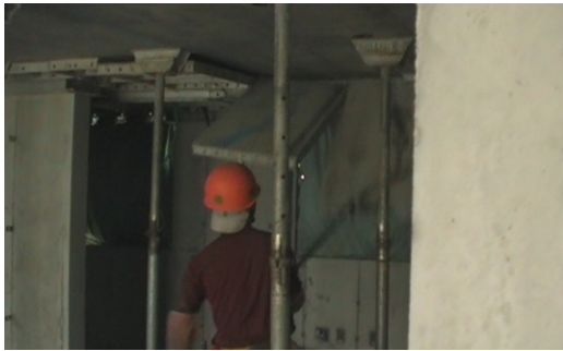
Fig. 7 Demolition work of gang form
