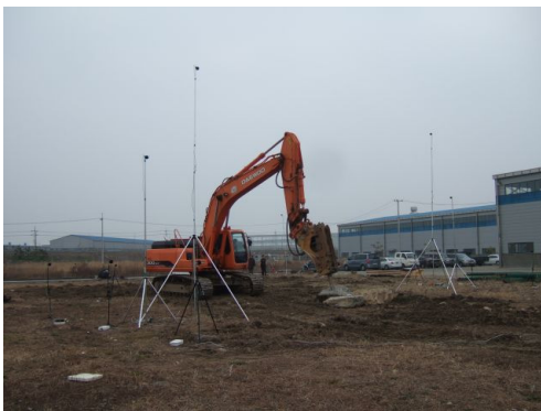
(a) Before installation
