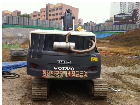
(b) After installation
