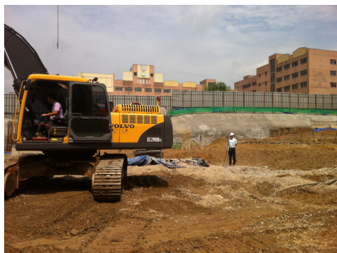
(a) Before installation
