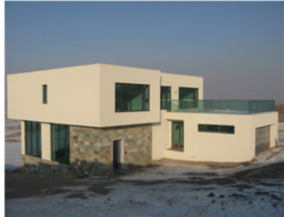
Fig. 1 Photo of residential building, where the vertical GHP system is installed.
