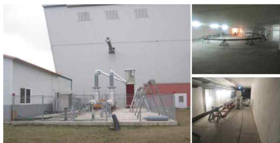
Fig. 3. Test setup in KEPCO Gochang testing fields [2]
