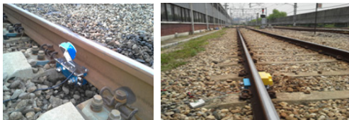
Fig. 3. Installation of the axle counter header
