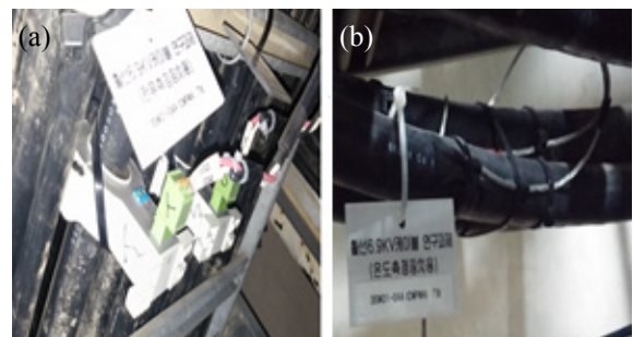
Fig. 3. Installation of the (a) current sensor and (b) temperature sensor.
