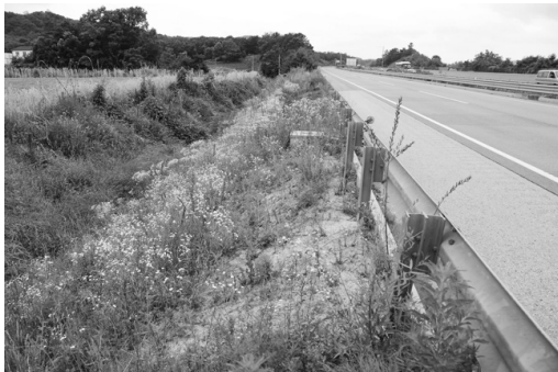
Figure 11. Monitoring of control test constructed (2015.8)
