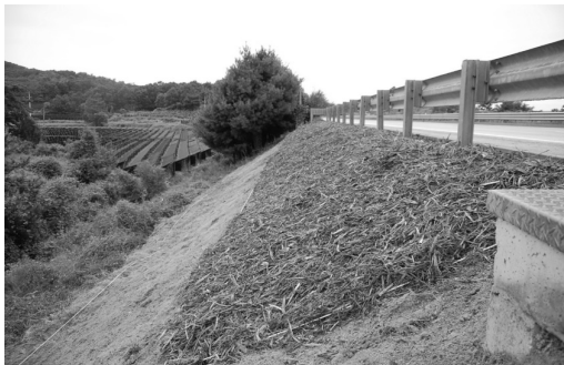
Figure 2. View of woodchip(100mm) test constructed (2013.9)
