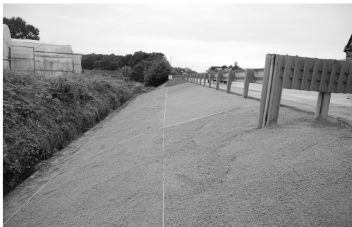
Figure 4. View of solidifying test constructed (2013.9)
