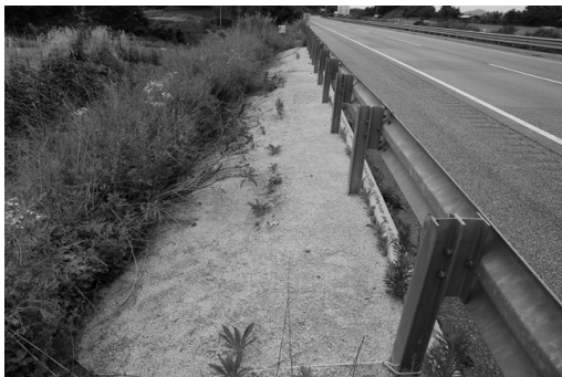
Figure 9. Monitoring of solidifying test constructed (2015.8)
