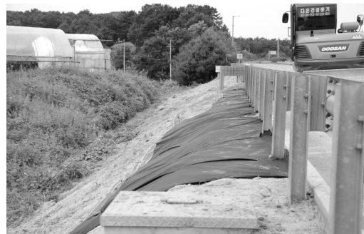
Figure 5. View of non woven fabric test constructed (2013.9)
