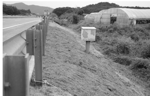
Figure 3. View of woodchip(50mm) test constructed (2013.9)
