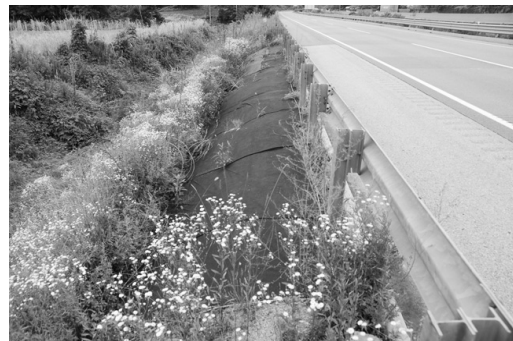
Figure 10. Monitoring of non woven fabric test constructed(2015.8)
