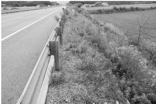
Figure 7. Monitoring of woodchip(100mm) test constructed(2015.8)
