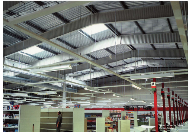
Fig. 2. Building structures of corrugated web girder
