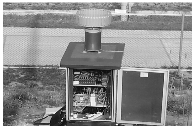
(b) Rainfall gauge
