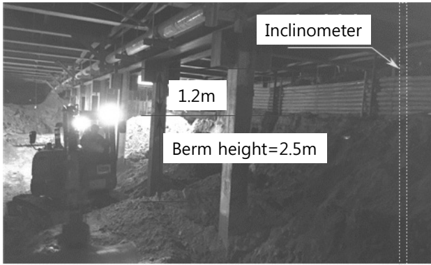
Fig. 2. Bermed excavation situation at the site
